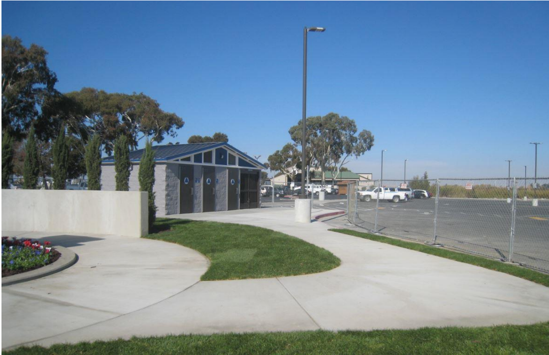
City Funded Path of Travel Between Restroom and War Memorial
