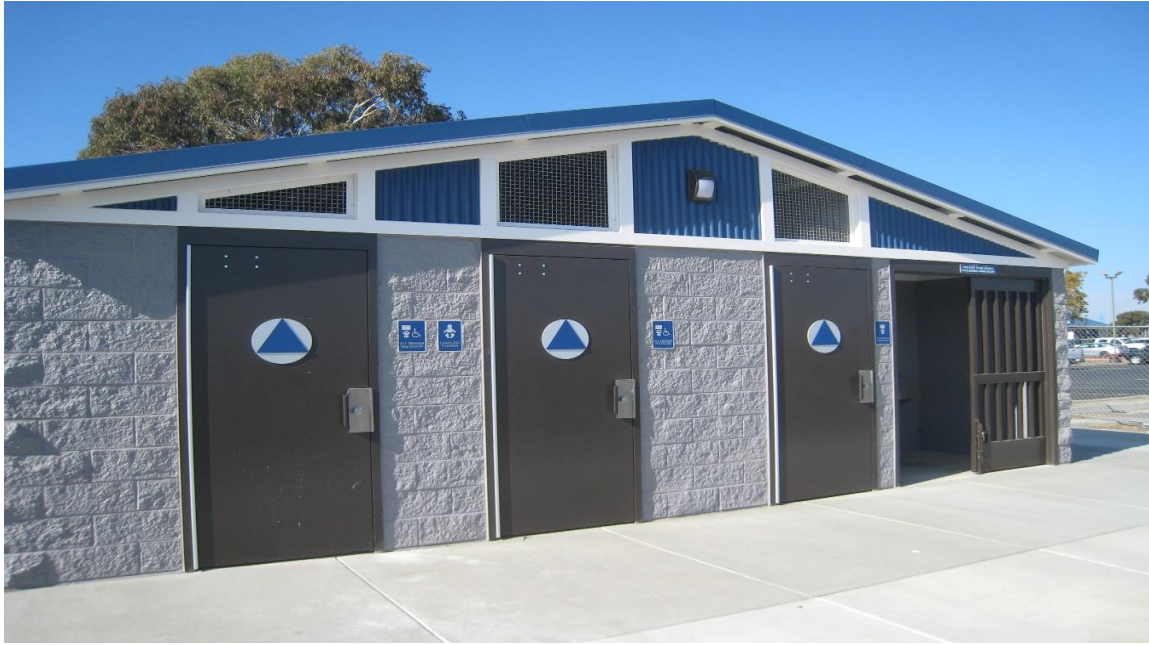
3 Unit ADA Compliant Restroom
