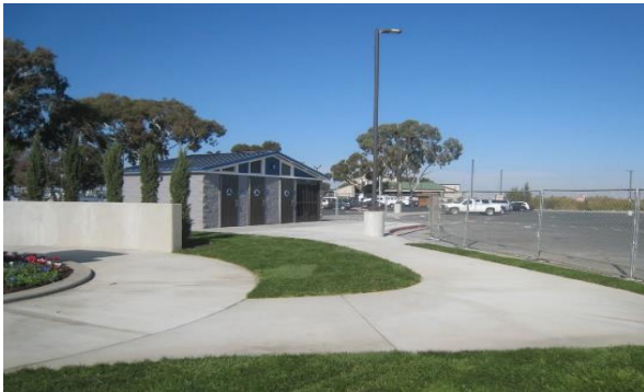
Restroom and Parking Area
